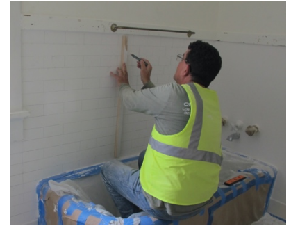
Plaster tiles in progress
