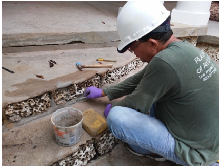
Stucco Repairs in progress
